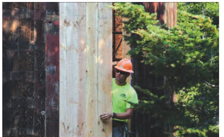
Cody Marks finishes the frame that will strengthen the tower.
